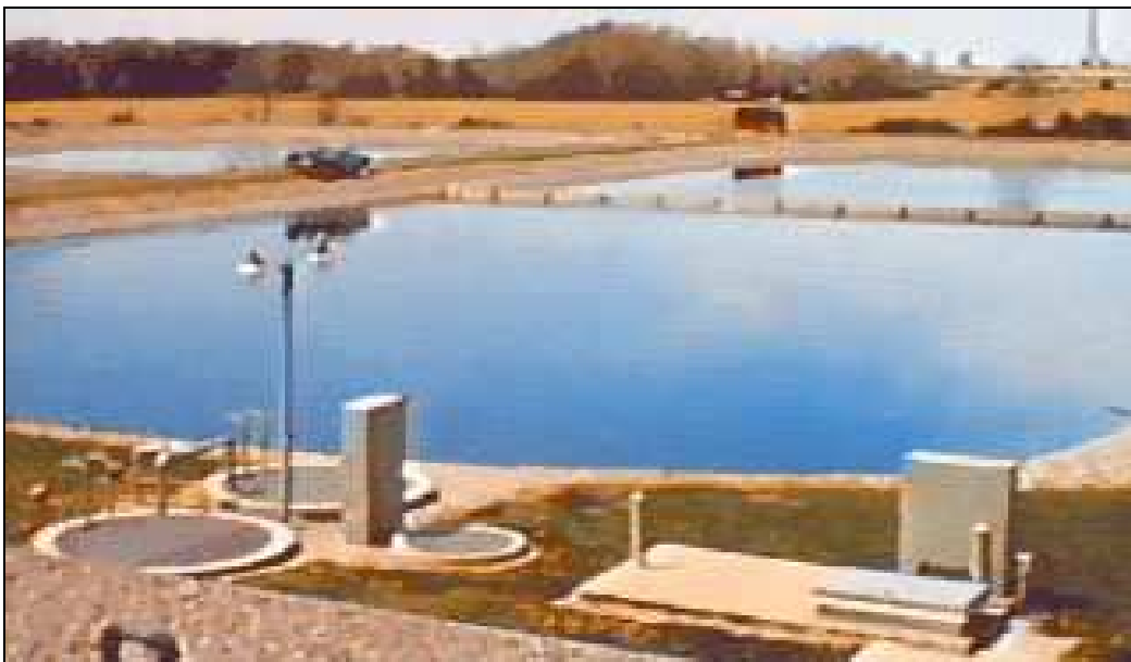
Figure 4. Photograph of a settling lagoon used for wastewater processing in a small municipality (Purdue 1999)
