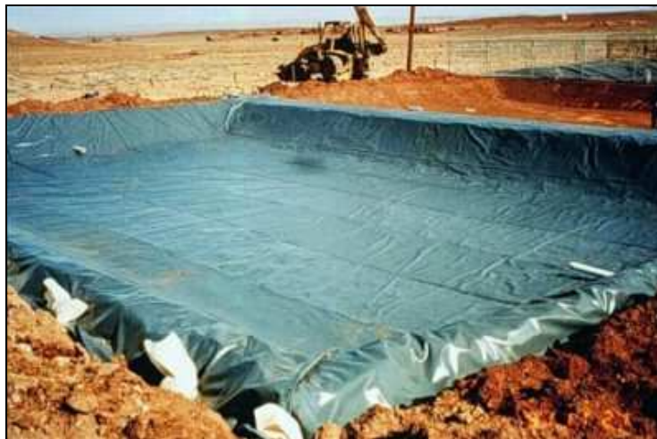
Figure 8. Construction site showing a synthetic plastic wetland liner (Purdue 2007)
